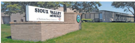
Sioux Valley Energy's headquarters, Colman, S.D.
