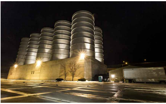
Surge tanks at Garrison Dam hydropower plant near Riverdale, N.D. The power plant has five generating units that produce an annual average 2.6 million mega-watt hours of electricity, valued in excess of $39 million in revenue.
